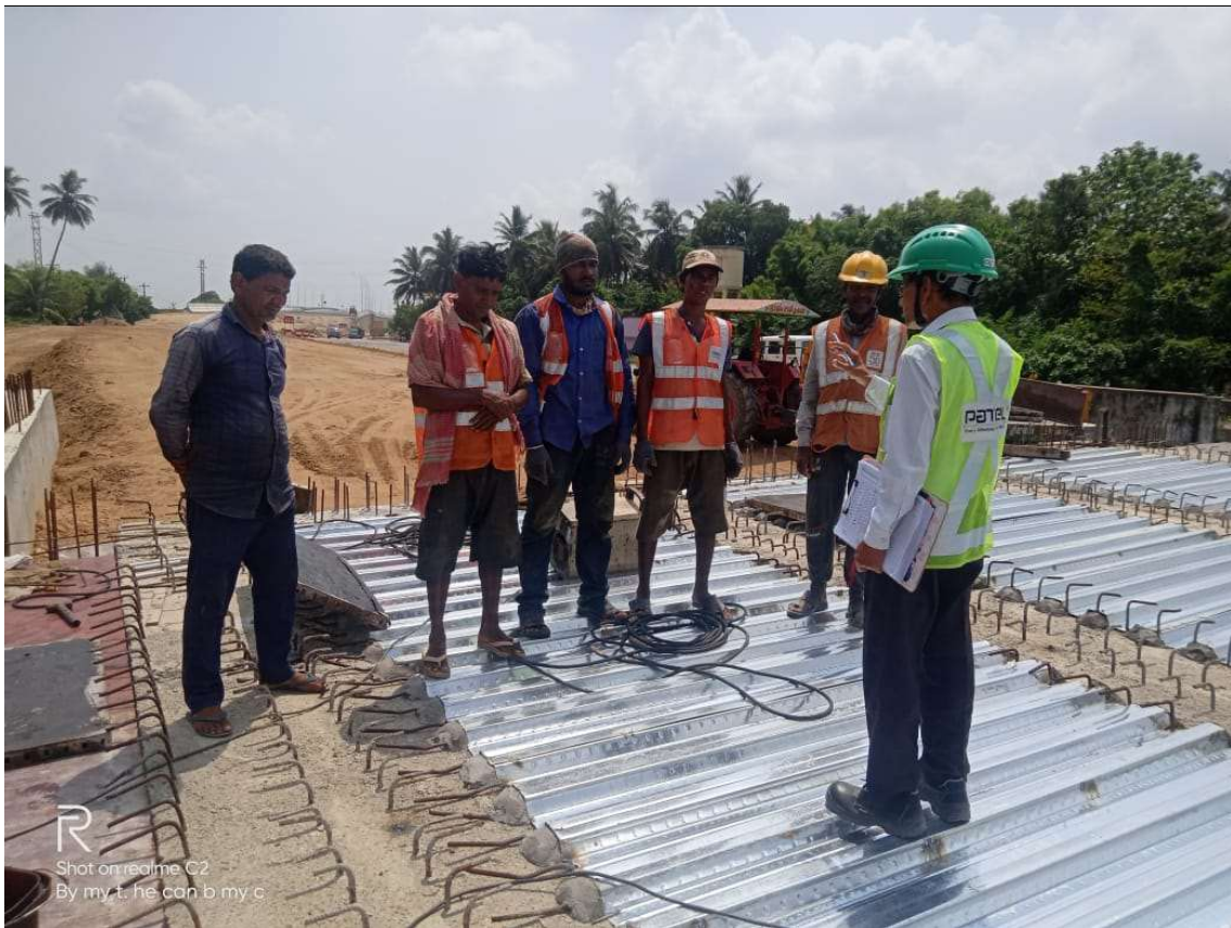
Safety instructions given to labours at Km.131+963 (Major Bridge)
